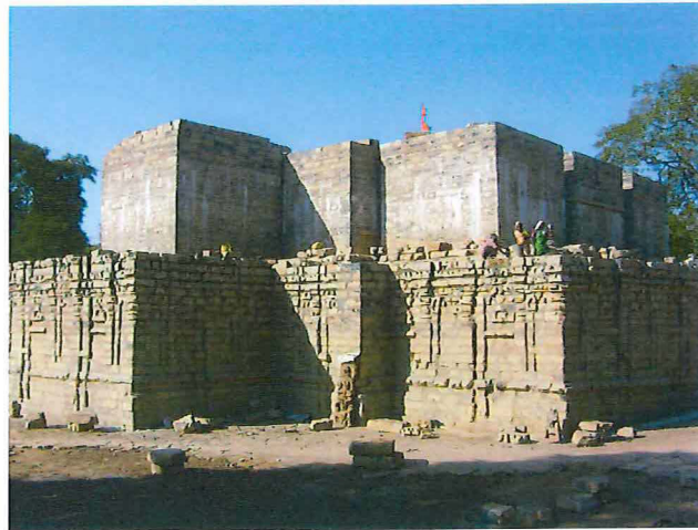
Plate 3.24: Backside of the Temple Construction
